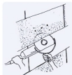
Preparation of the cut for the semi-cylindrical and circular segment flat jacks using a cutting saw
