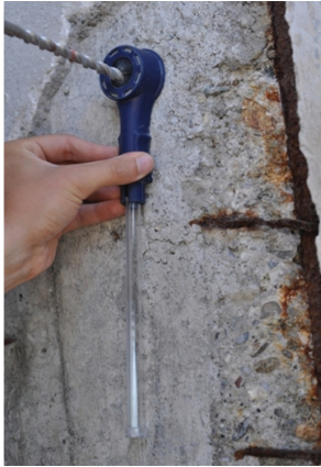
Drilling phase with powder collection for carbonation test
